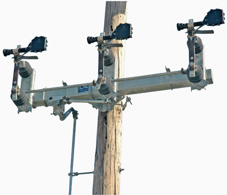
Vertical (Riser) Configuration
